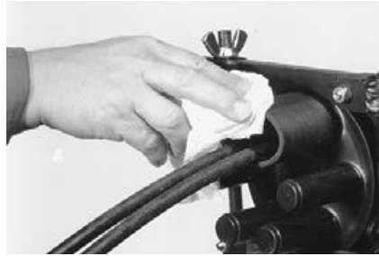
6.1 Thoroughly clean oval port and cable sheath with the cleaning tissue over a distance of 100 mm from the edge of the port.
