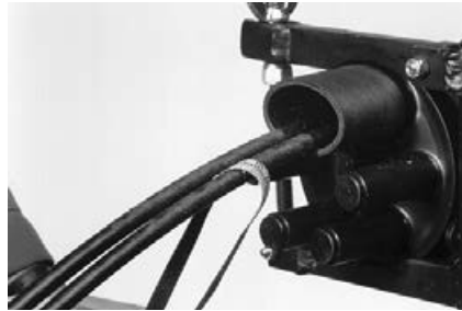
6.2 Abrade oval port and cable sheath circumferentially on the cleaned area with the abrasive strip. Remove any abraded material with a clean cloth.
