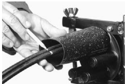
6.3 Place oval seal over the oval port and cable. Mark the sleeve length onto the cable.
