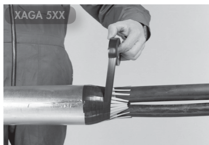
9 Using PVC tape (not included in standard kit except for XAGA 530), tape the crowns, starting from the liner/canister body (10 mm), down to the cables with a 50% overlap.
