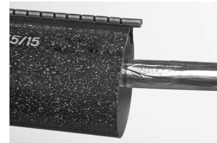
16 Center the sleeve between the blue lines of the aluminum cable foils.
