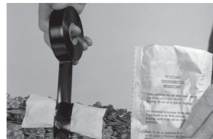
6 Take the desiccant out of the aluminum bag and place it within the joint.
